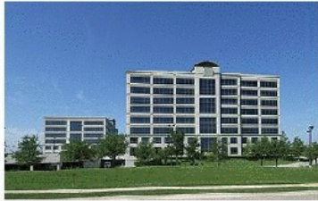
Las Colinas Corporate Center I & II 6363 North State Hwy. 161 Irving, TX
