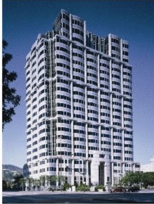
Nestle 800 North Brand Boulevard Glendale, CA
