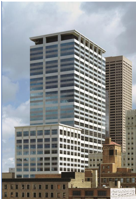
US BANCORP CENTER, MINNEAPOLIS
