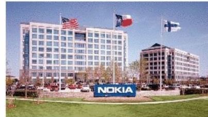
6011 & 6021 Connection Drive Irving, TX
