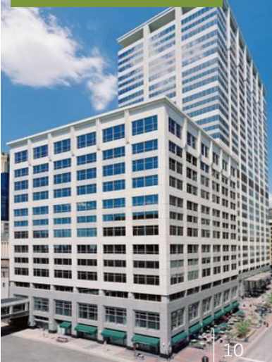
US Bancorp | Built 2000
