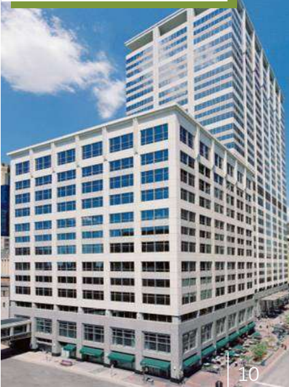
US Bancorp | Built 2000
