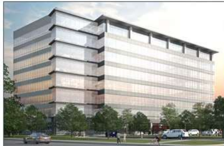
Connection Drive, Dallas 500K SF
