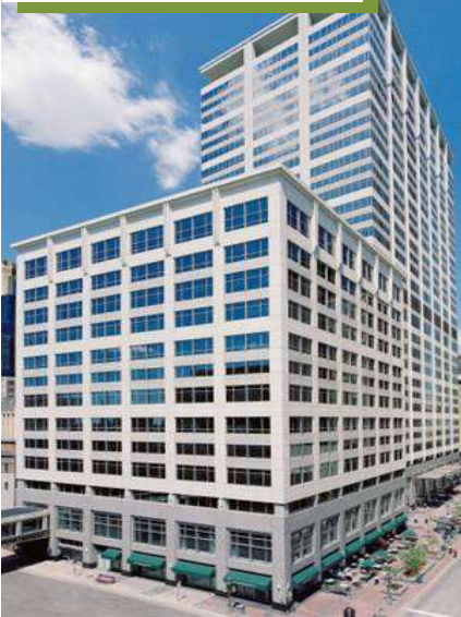
US Bancorp | Built 2000
